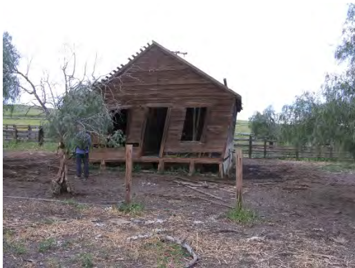
Figure 15: P-39-000120 (Update), Three room structure overview
