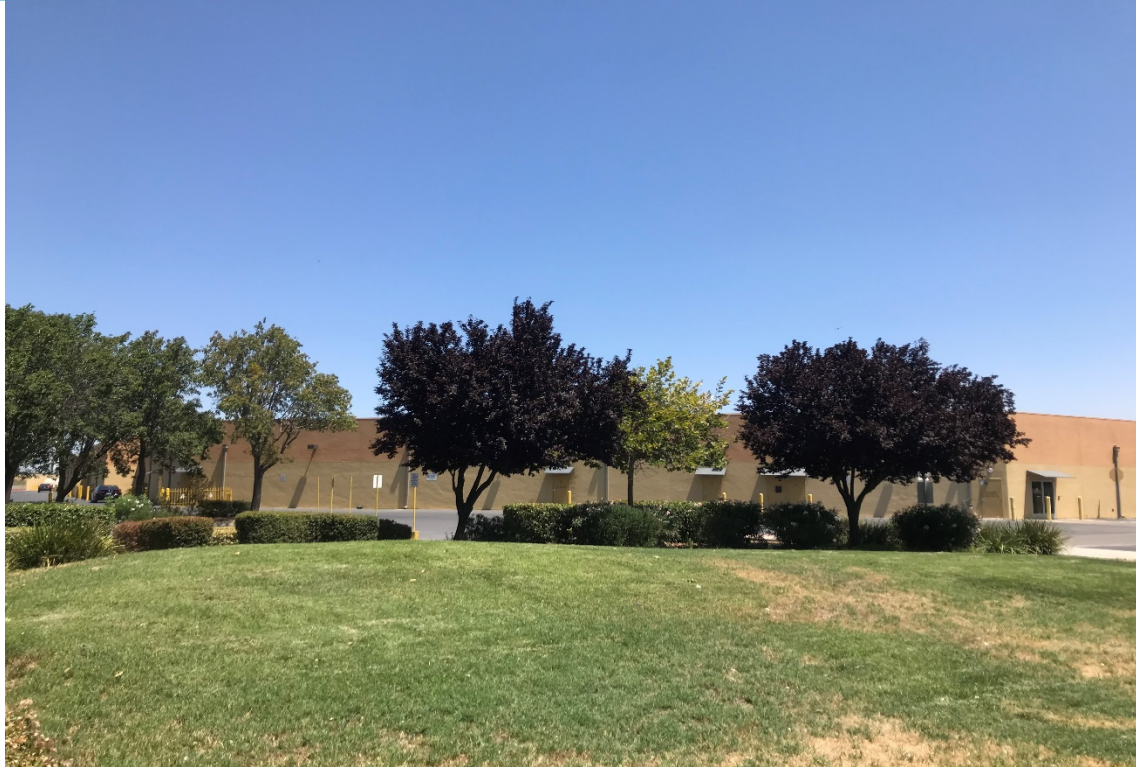
Photograph 1: Overview from the southwest corner of the project site; facing northeast.
