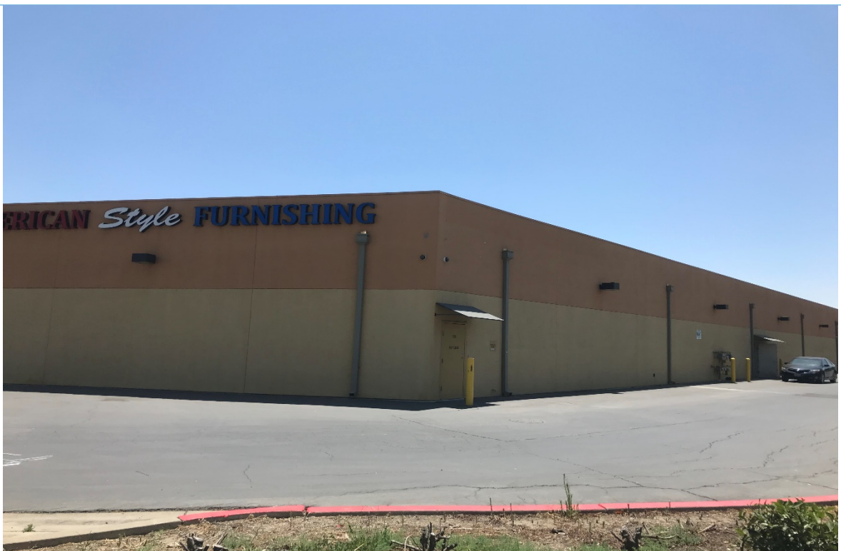
Photograph 2: Overview from the northwest corner of the project site; facing southeast.
