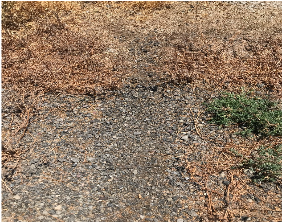
Photograph 6: Representative soil composition of the project site.
