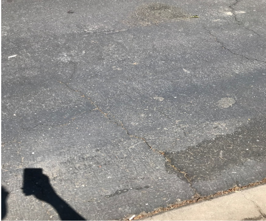
Photograph 7: Representative composition of the hardscaped surface of the project site.
