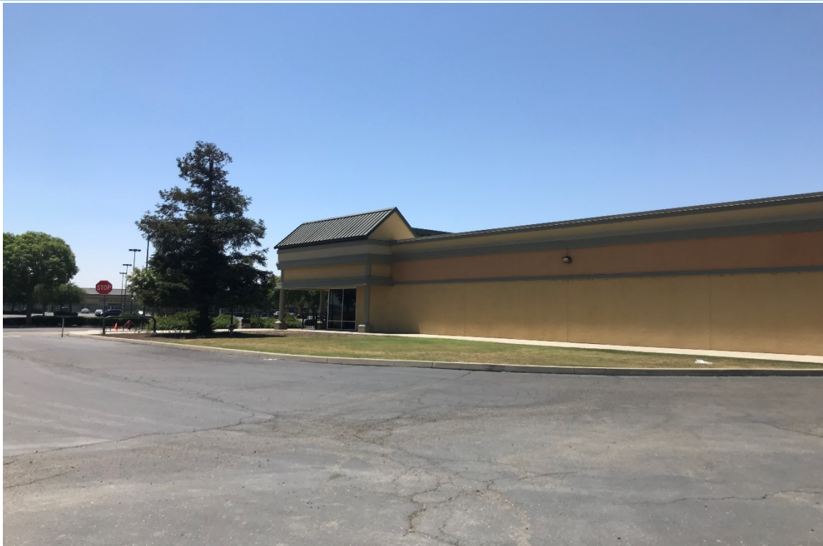
Photograph 3: Overview from the northeast corner of the project site; facing southwest.
