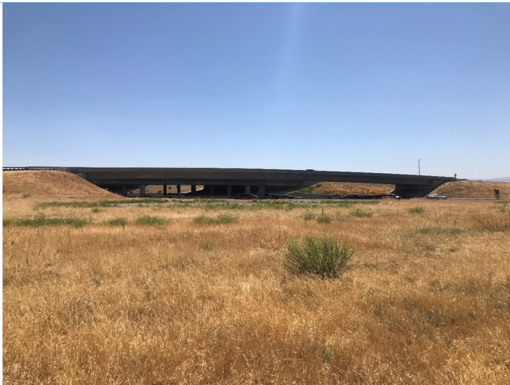
Photograph 2: Overview from the northwest corner of the project site; facing southeast.
