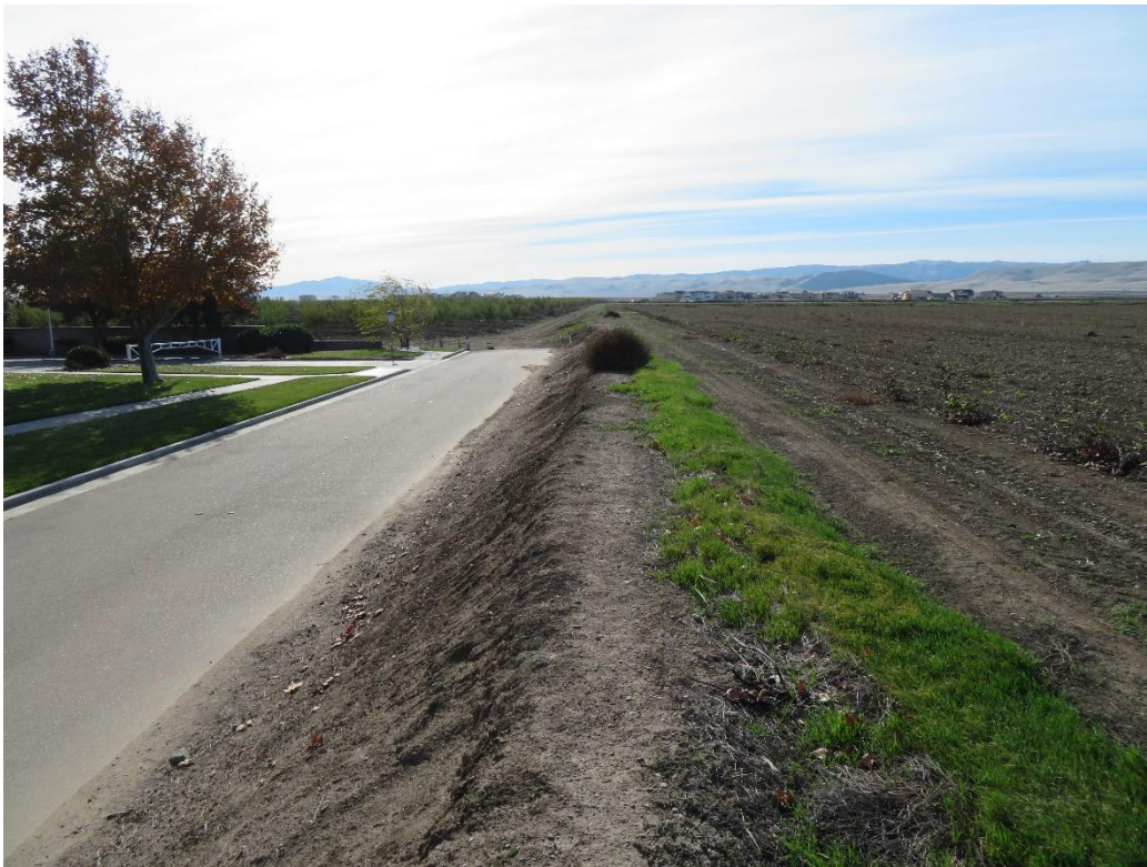
Photograph 6: Looking south along the eastern boundary of the project site.
