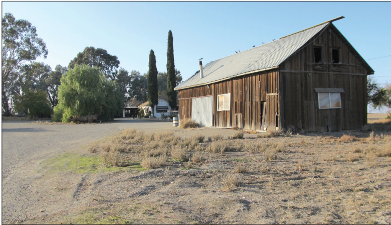
4.1-2a: View of the Residence at 24383 Mountain House Parkway
