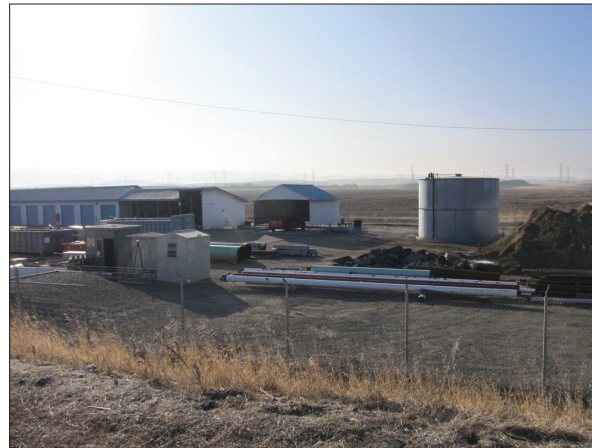
4.1-2d: View of the Pacific Gas & Electric Facility from the Off-Ramp of Interstate 205
