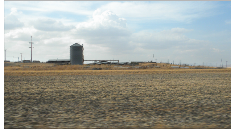
4.1-2b: View of the Cell Tower Installation Facilities from Mountain House Parkway
