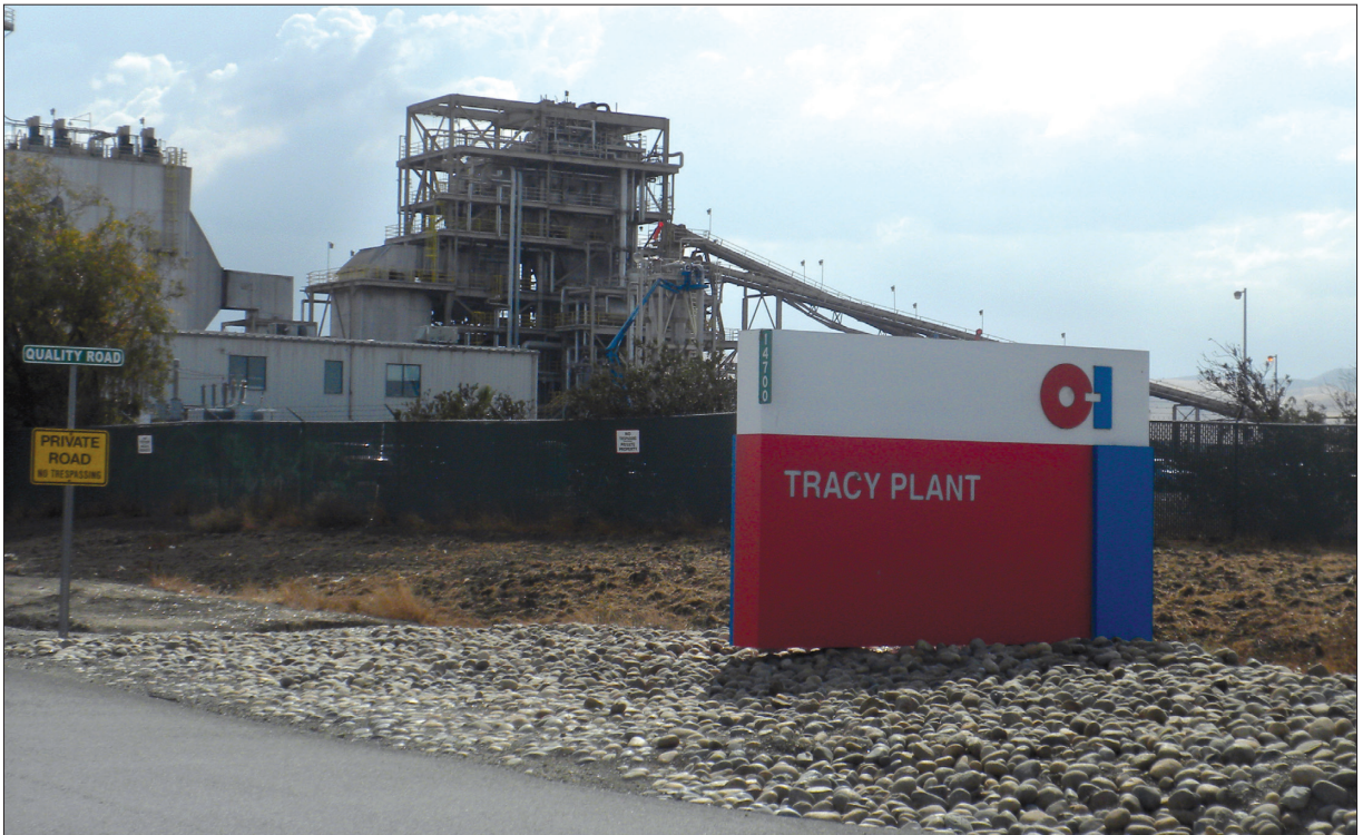
4.1-3b: View of the Tracy Biomass Plant
