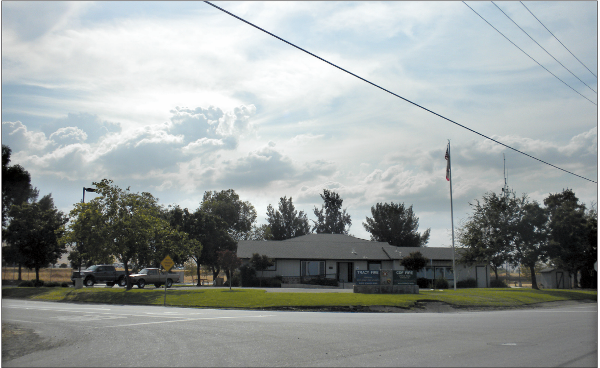
4.1-3a: View of South County Fire Authority Station 94/California Department of Fire Station 26
