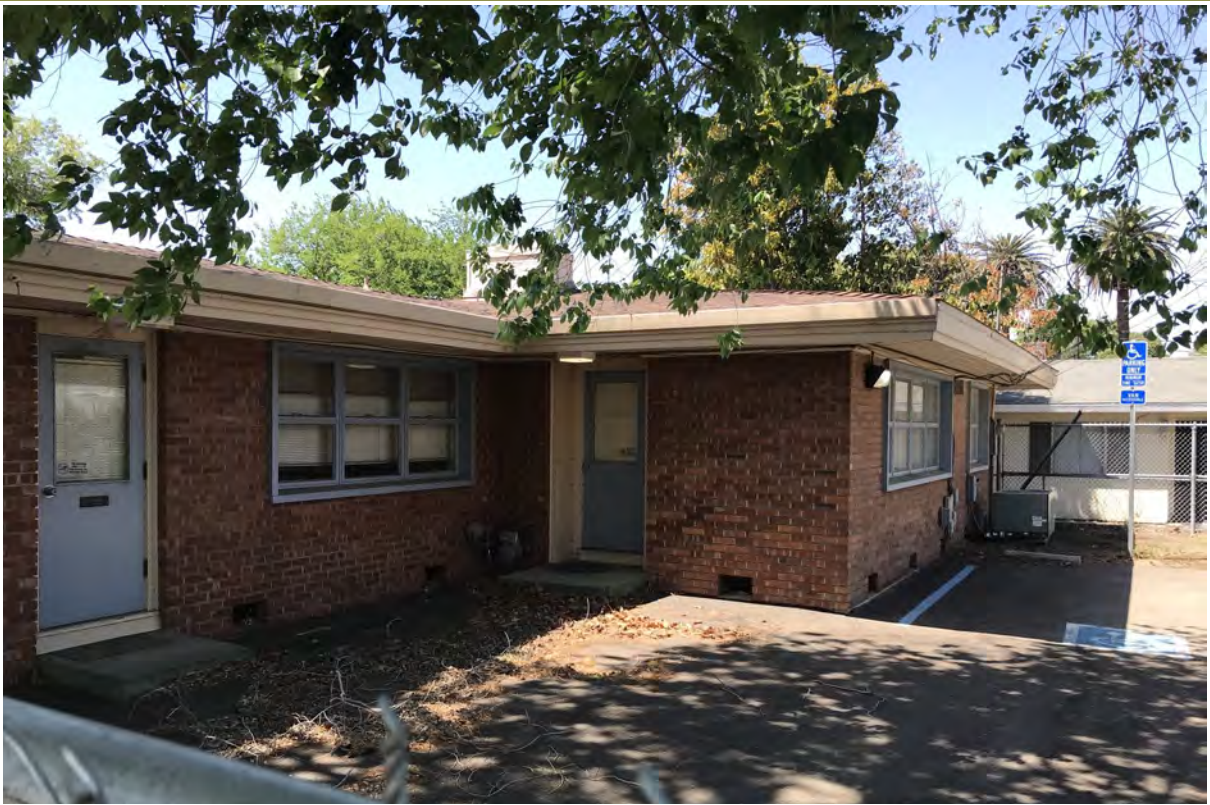
1- NORTHEAST REAR OF BUILDING
