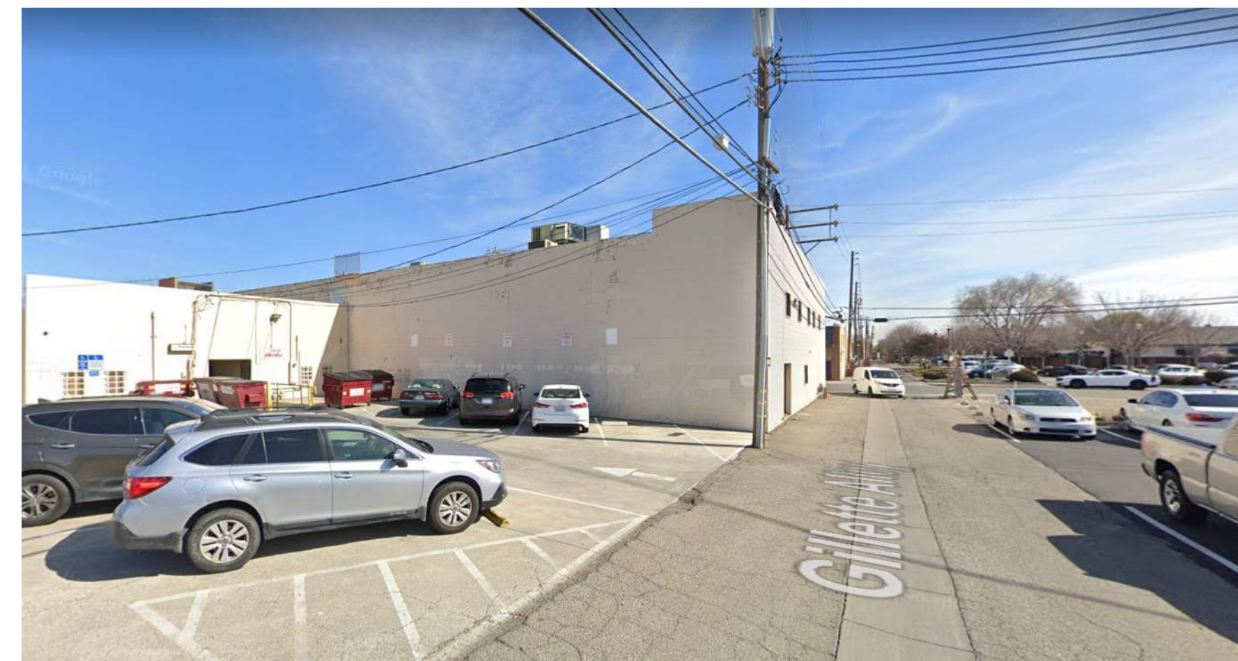
9 VIEW EAST DOWN GILLETTE ALLEY, BUILDING ON LEFT (MIDDLE OF IMAGE)
