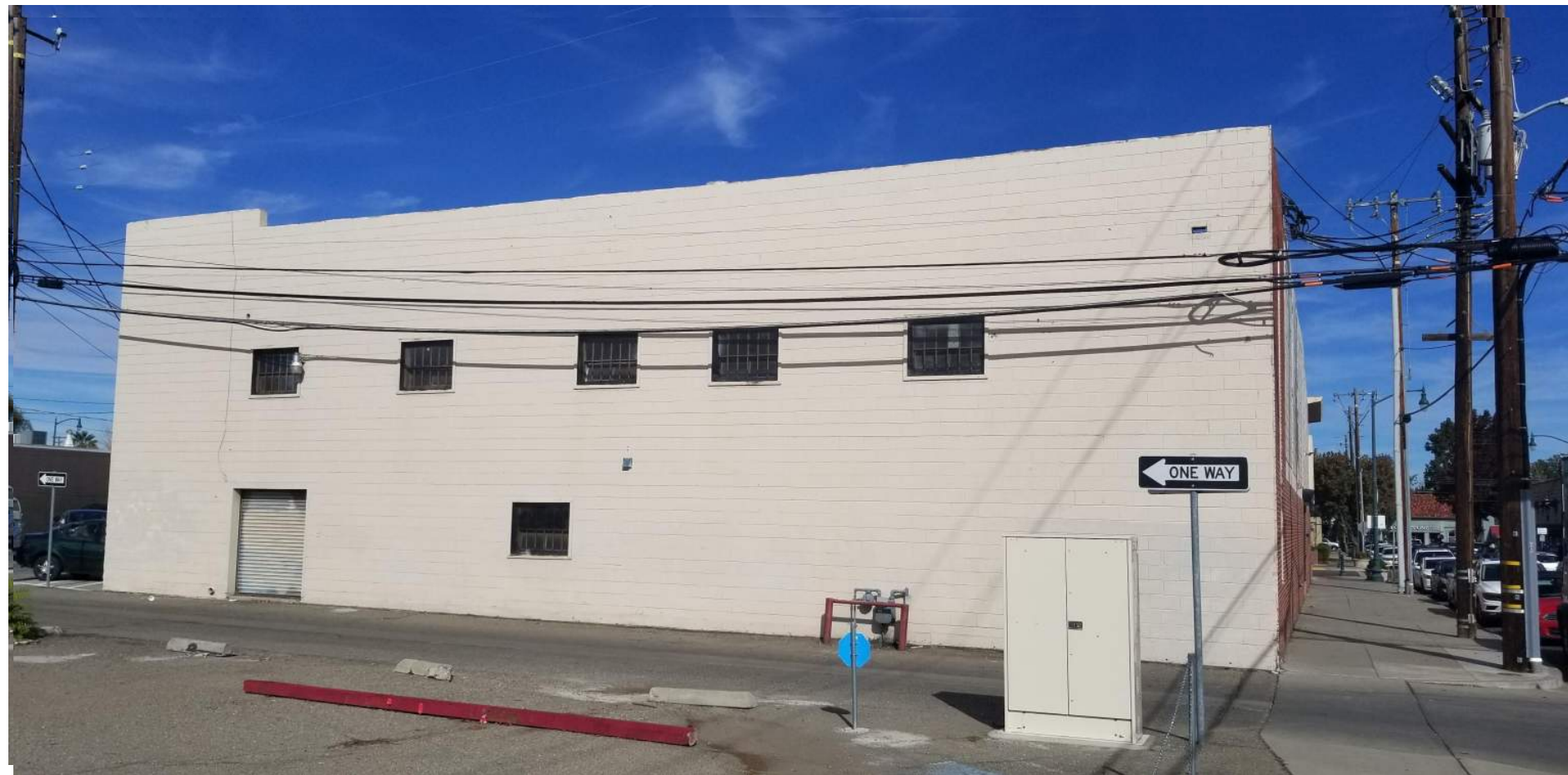
1 SOUTH ELEVATION FROM ALLEY
