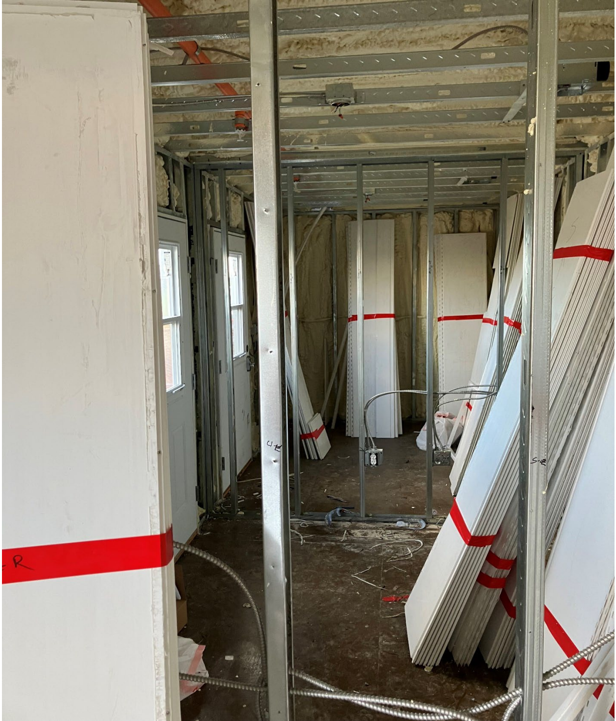
Figure 3-4 Photos 3 and 4: Shows frame exposed from removal of paneling.
