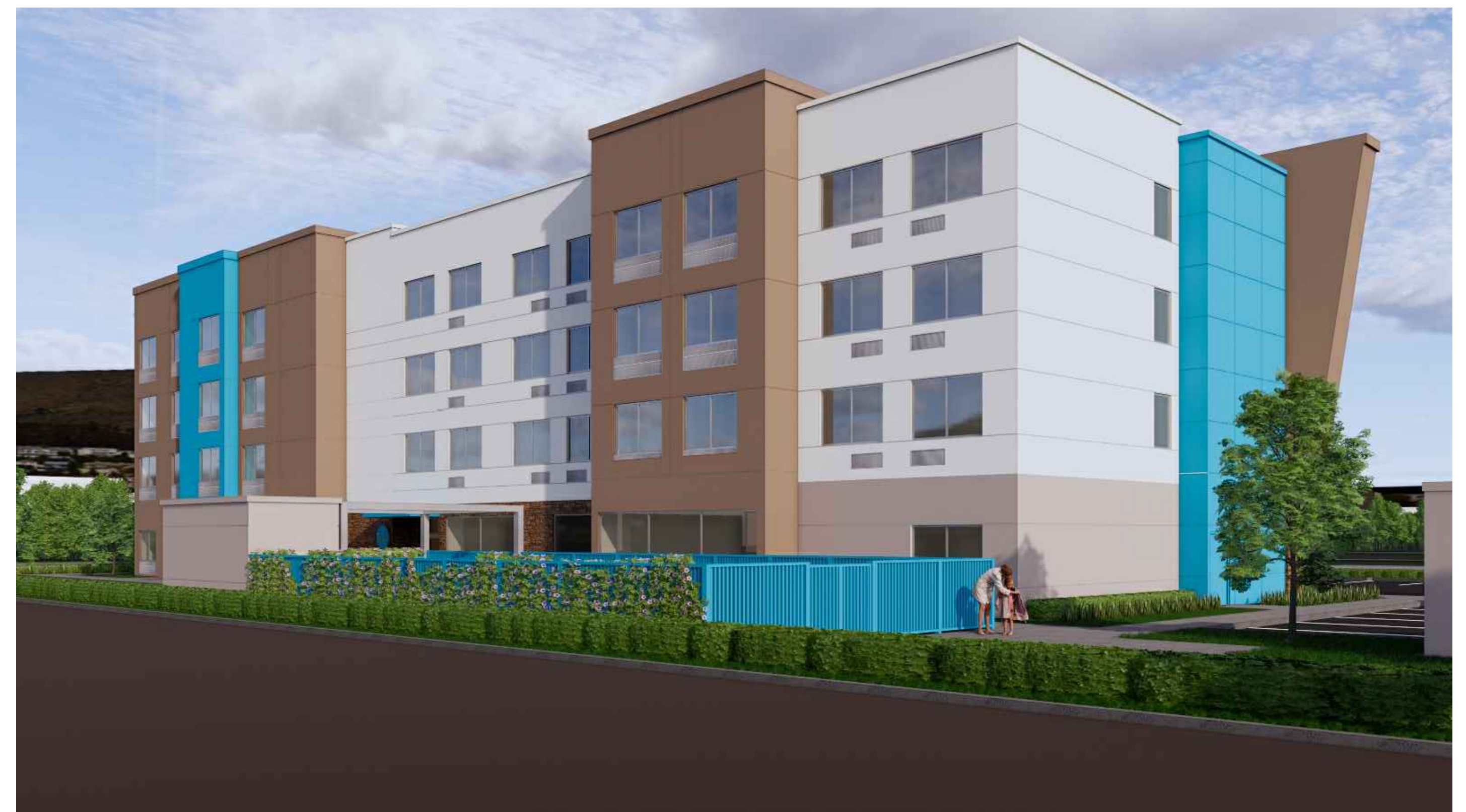
4 STREET VIEW LOOKING NORTH-EAST
