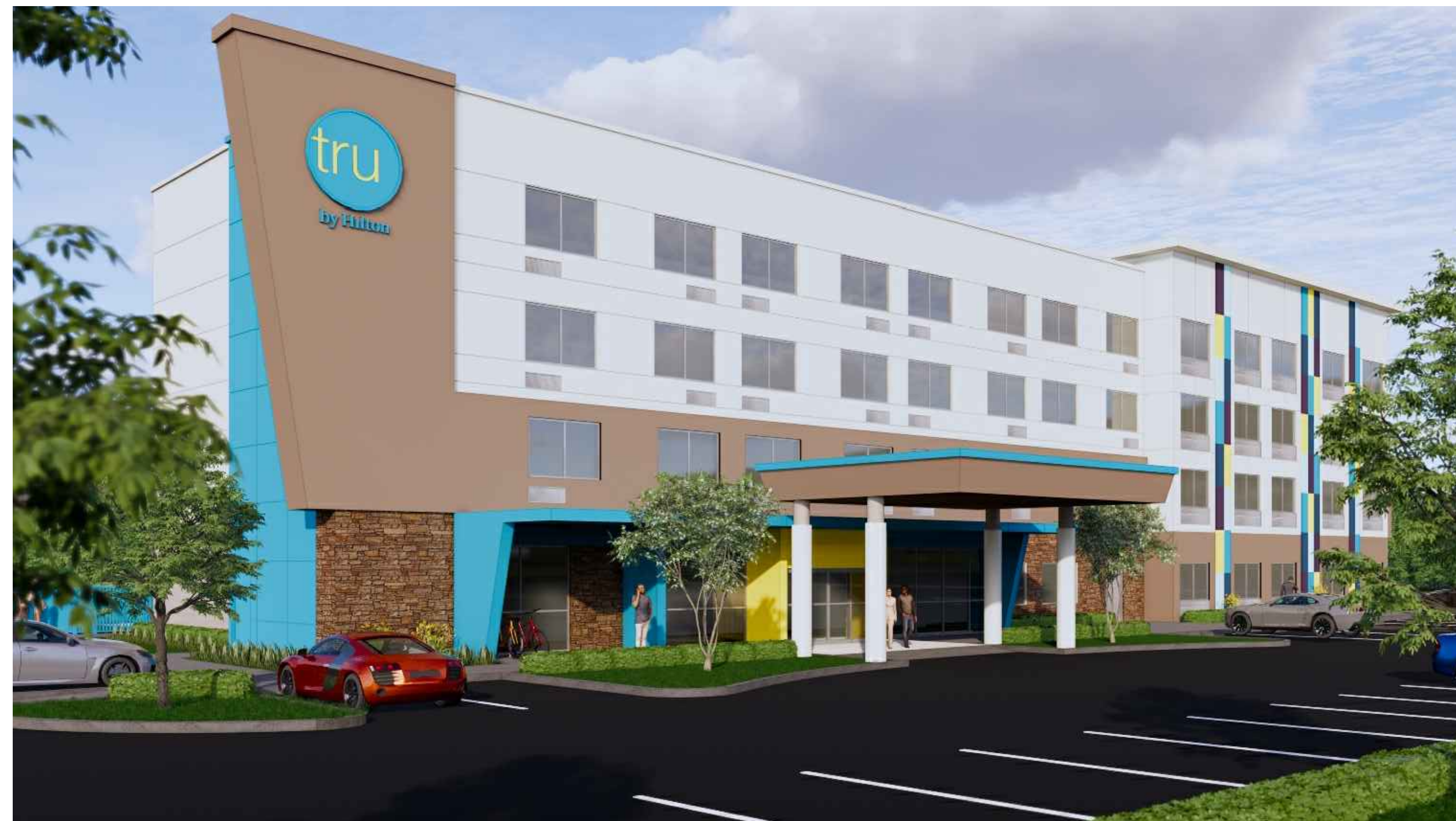
1 STREET VIEW LOOKING NORTH-EAST
