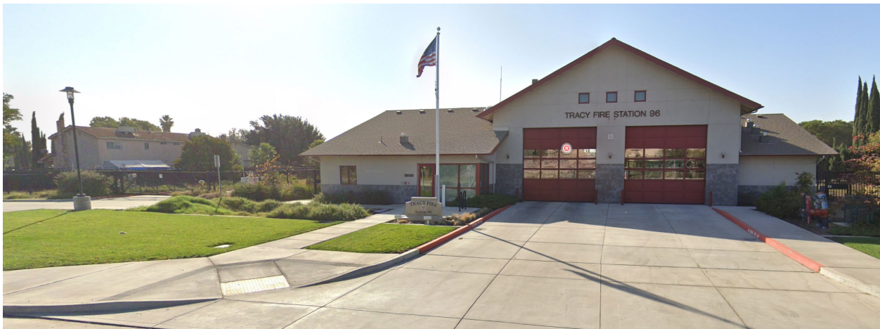
Figure 34 – 2014 Tracy Fire Station 96, 1800 West Grant Line Road (to remain)
