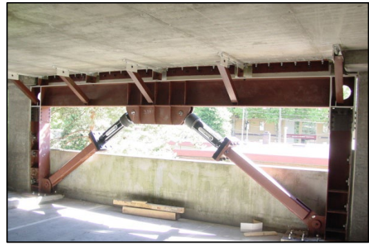
Figure 55 – Viscous Damper Retrofit, Kent WA
