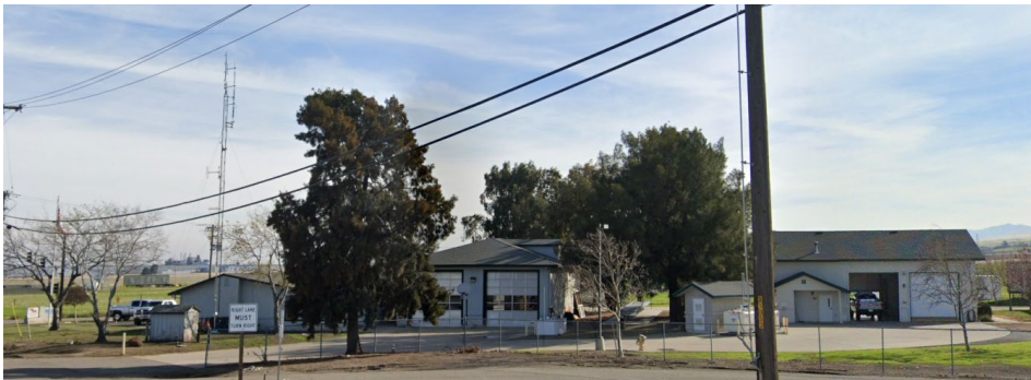
Figure 9 – 1995 Tracy Rural Fire Station 94, 16502 West Schulte Road (to be relocated)
