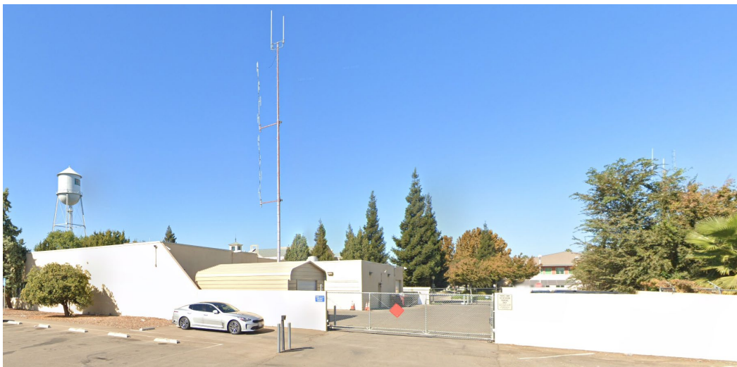
Figure 41 – Back of 1979 Tracy Police Building, 400 East 10th Street (to be demolished)
