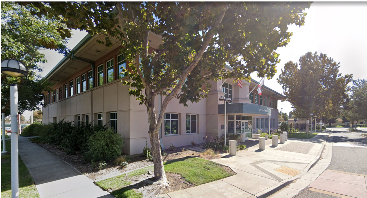
Figure 39 - 1996 Tracy Police Department, 1000 Civic Center Dr (to receive tenant improvement & addition)
