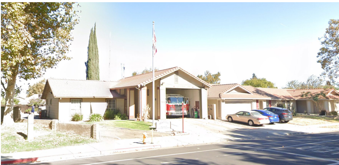
Figure 10 – 1986 Tracy Fire Station 97, 595 West Central Ave (to be relocated)
