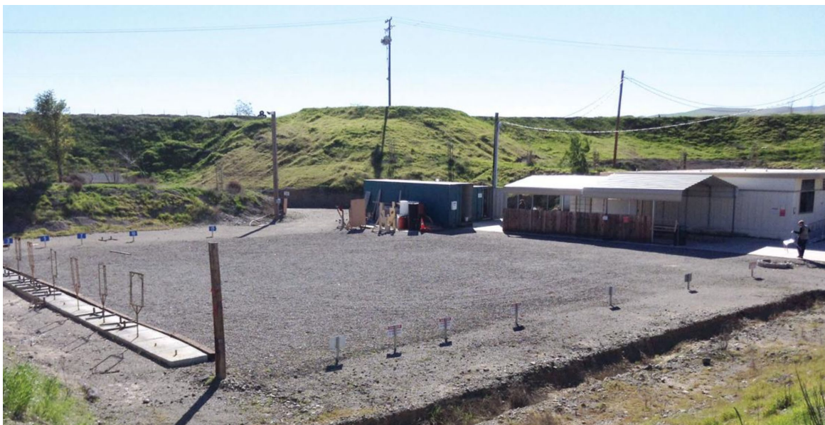
Figure 51 - Captain John J. Serpa Memorial Police Training Facility (to be upgraded and expanded)
