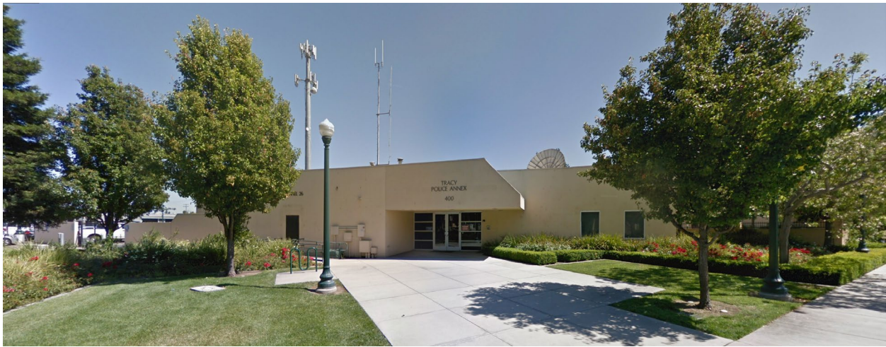
Figure 38 - 1979 Tracy Police Building, 400 East 10 th Street (to be demolished)
