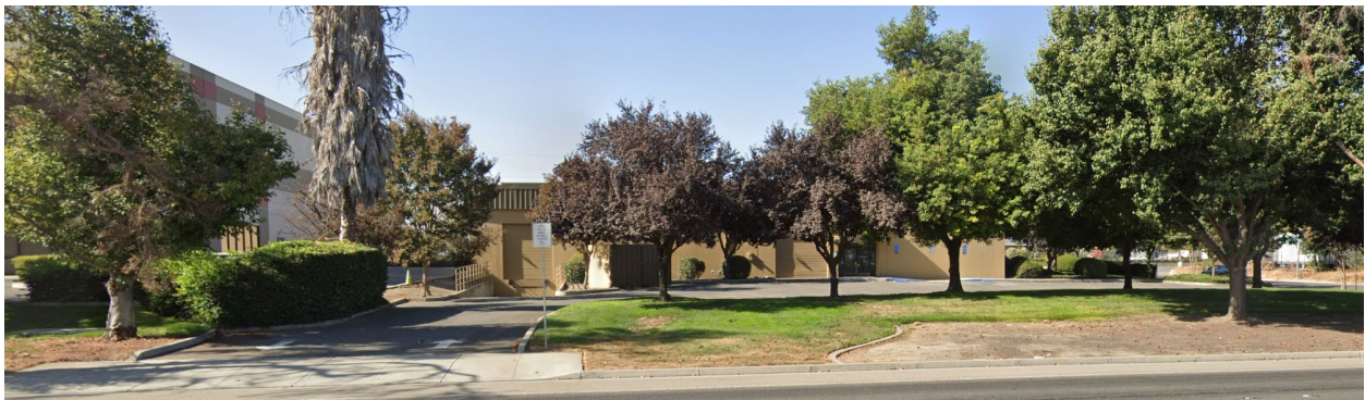
Figure 50 - Leased North Annex Space, 1325 North MacArthur Drive (to be let go)
