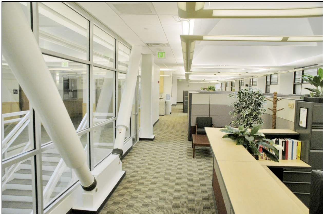
Figure 61 - Earthquake Protected Police Building with Seismic Dampers & Daylighting, Vacaville, CA
