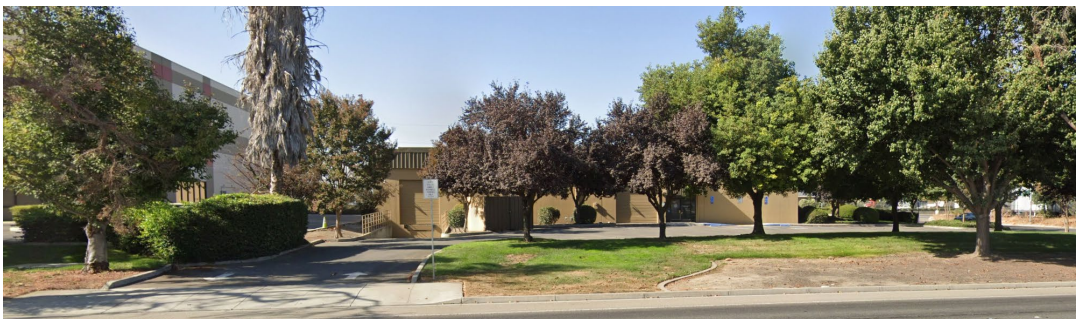
Figure 12 - Leased North Annex Space, 1325 North MacArthur Drive (to be let go)
