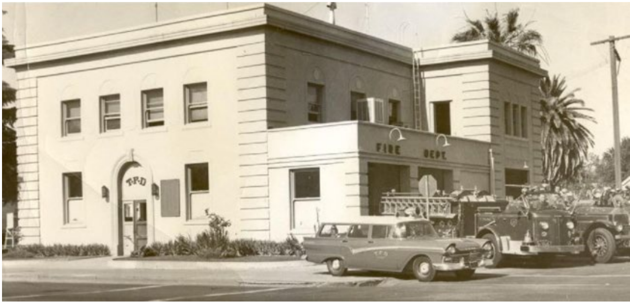
Figure 24 – 1916 Tracy Fire Department Building, 835 Central Avenue (to be upgraded)
