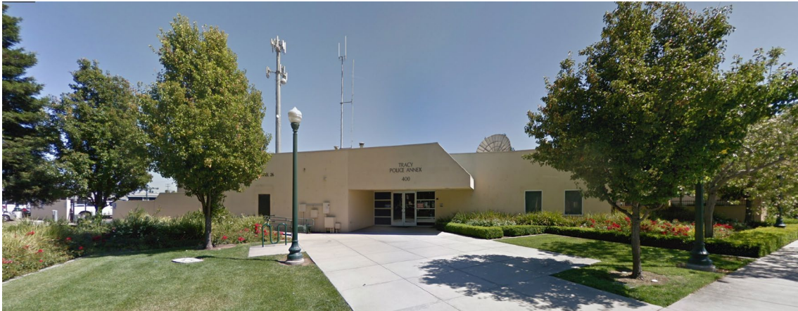
Figure 11 - 1979 Tracy Police Building, 400 East 10 th Street (to be demolished)
