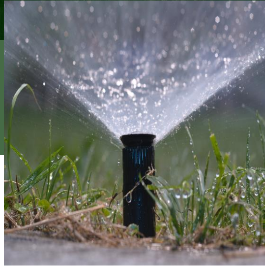
RECYCLED WATER PIPELINE
