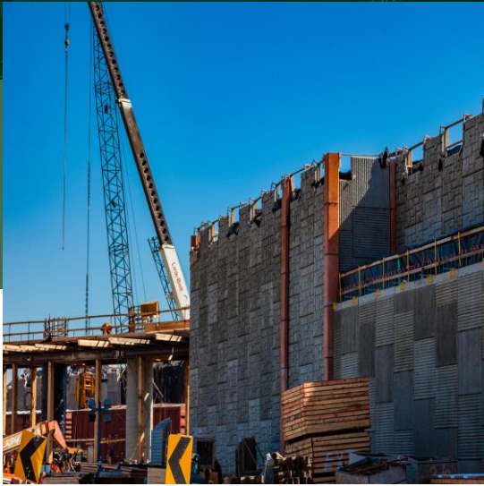
11 TH STREET BRIDGE REPLACEMENT
