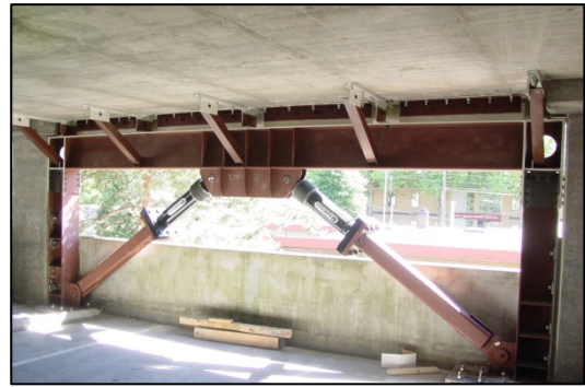
Figure 28 – Viscous Damper Retrofit, Kent WA
