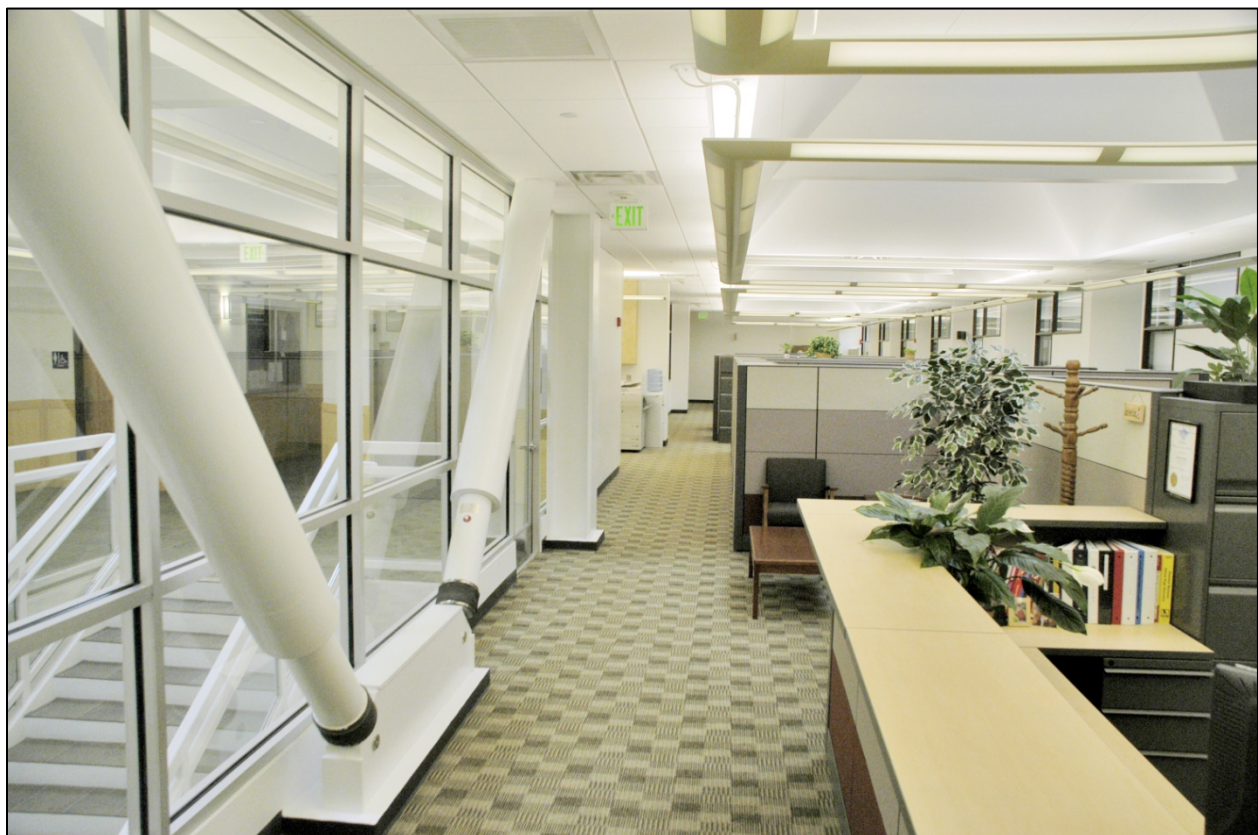
Figure 34 - Earthquake Protected Police Building with Seismic Dampers & Daylighting, Vacaville, CA
