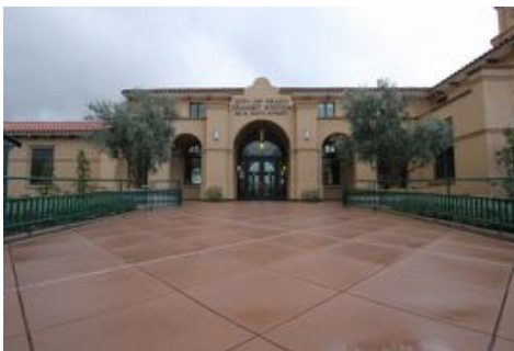
Tracy Transit Station, 6th & Central CIP77519
