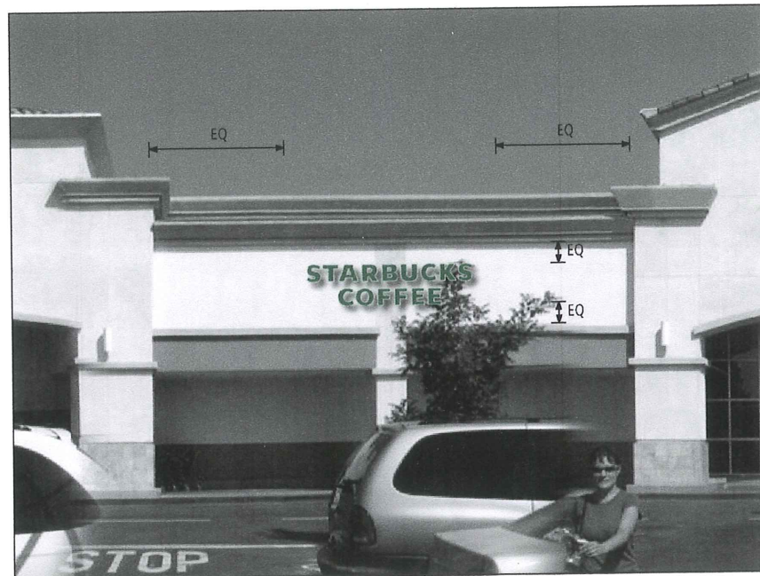
Right Fascia of Front Elevation
