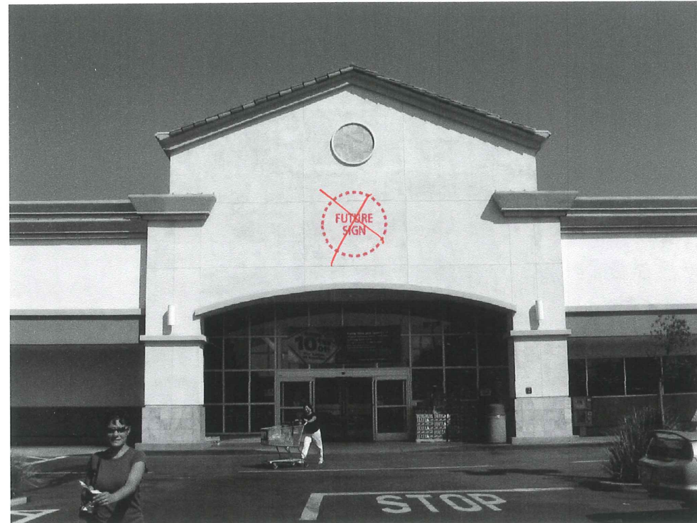
Right Tower of Front Elevation
