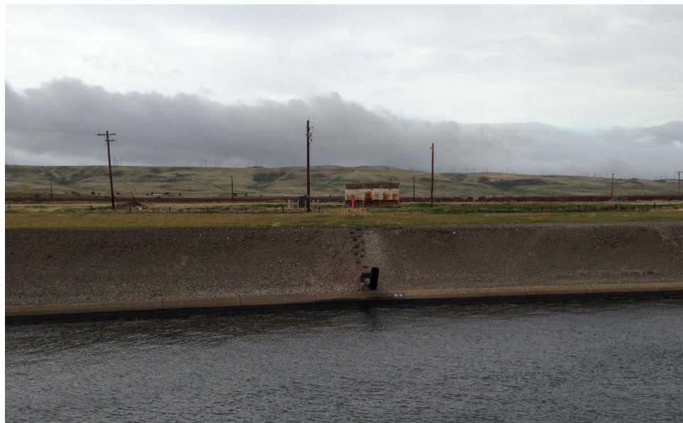
Photo 2. Taken from the east side of the Delta-Mendota Canal looking west, at canal mile 15.11. Shows a groundwater well discharge.
