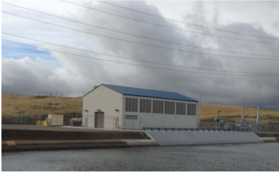
Photo 1. Taken from the east side of the Delta-Mendota Canal looking west, at canal mile 7.25. Background shows completed DMC intertie to California Aqueduct.
