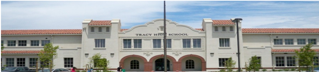
Tracy High School Classroom Building
