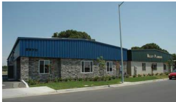
Poor building articulation, indistinguishable entrance,
