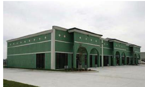
Obtrusive color, lack of windows, minimum landscaping
