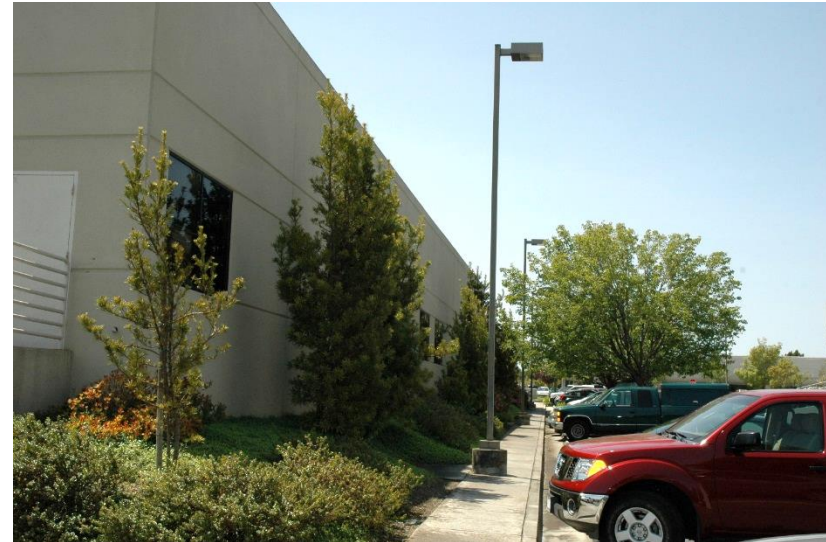
Discouraged lighting: Lighting pole blocking pedestrian walkway.
