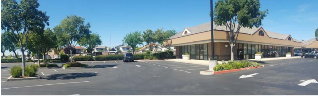
Image 1. Existing building and proposed play area location
