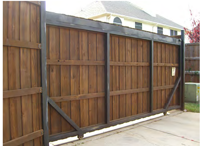
Figure 3.47 Eight-foot rolling gate
