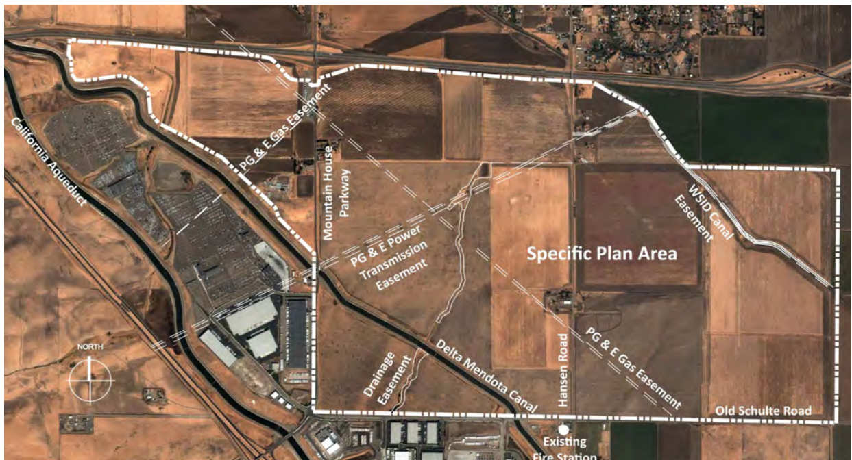
Figure 1.1, Site Aerial Photo
