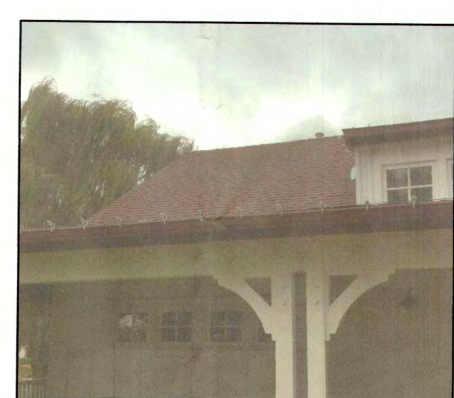
Asphalt Shingle Roof
