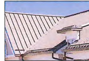
The Garland Company Standing Seam Roof
