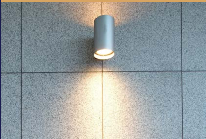
Exterior Lighting Is Installed To Enhance Safety Around the Area
