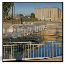
**Description**: The Selector comprises an unaerated section. Mixers are needed in absence of air to keep the solids afloat, and also
