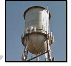
Description: Renovation of this historic tower is necessary to protect against corrosion. The foundation requires reinforcement and the existing steel components require repair & protection from corrosion. The Tower is historical, but not part
